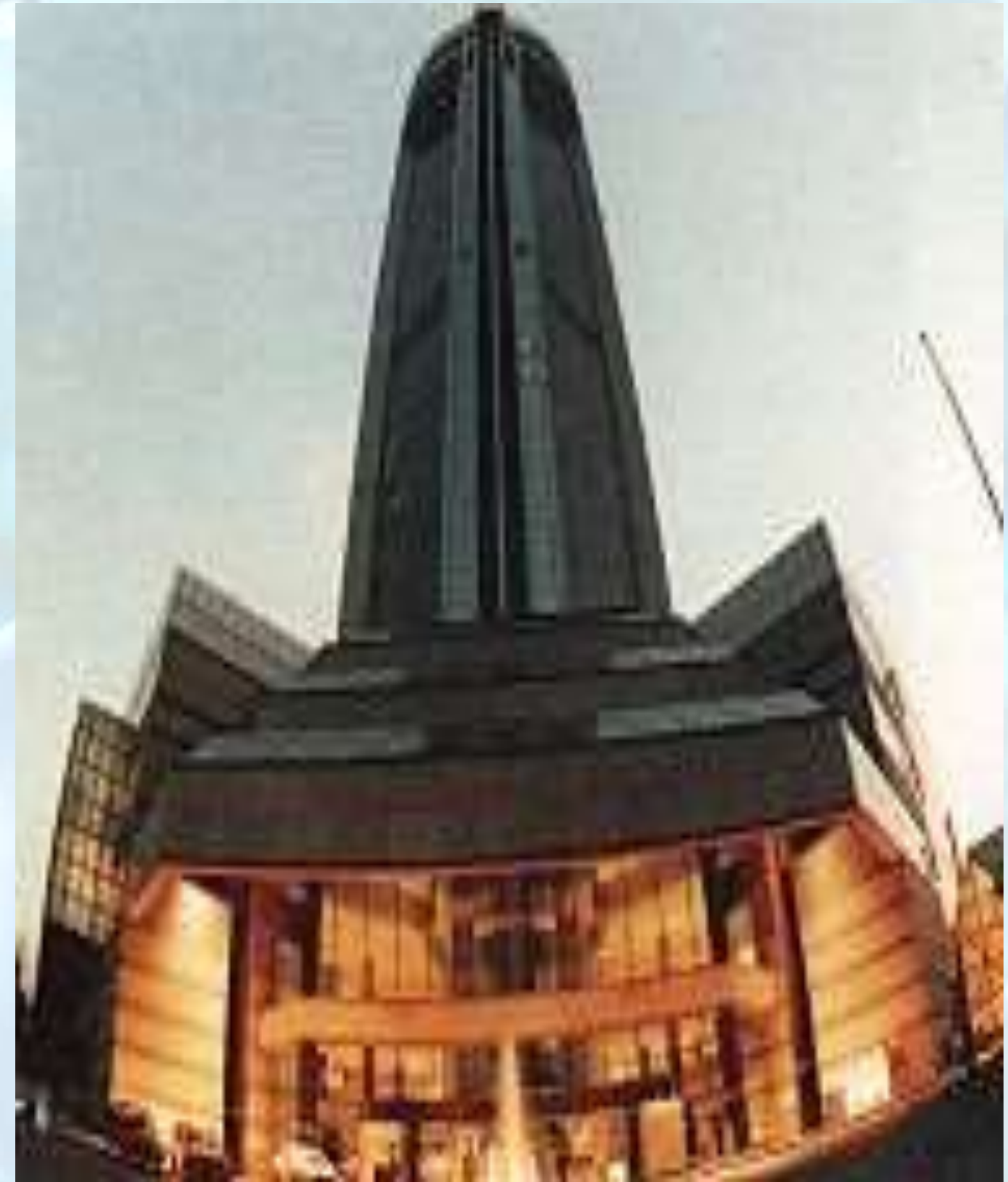
320,000 - GPD Bio-Pure (ACT) System constructed in the basement of the Jin Jiang Hotel and Commercial Center in Shanghai, China
